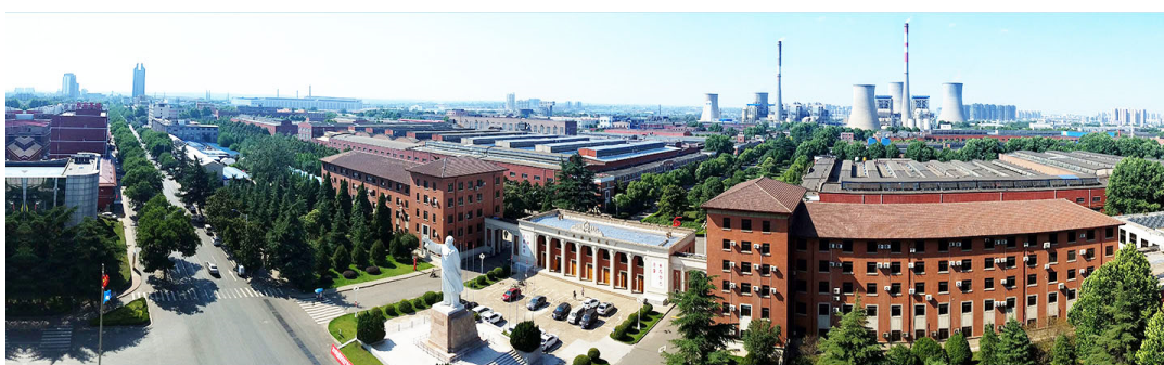
Figure B1. Contemporary view of the Luoyang Truck Factory.
